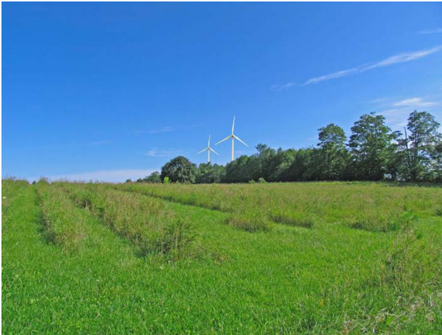
View 4 – Looking Northeast from the corner of 8 th Concession and Artemesia-Osprey Townline at Turbines #1 and #2
