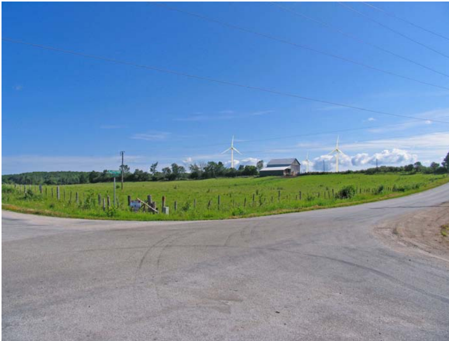
View 7 – Looking Northeast from the corner of 8 th Concession and 35 Sideroad at Turbines #3, #4, and #5
