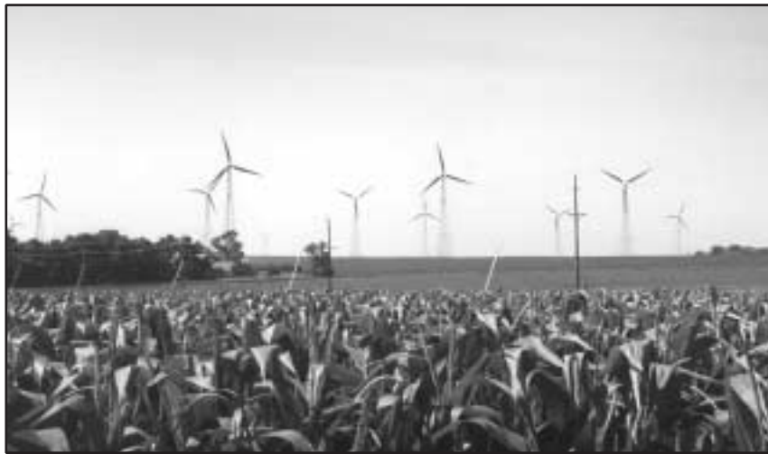
FIGURE 7.1 750 kW ZOND WIND TURBINES 1.5 MILES EAST OF ALTA, IOWA PHOTO COURTESY: WAVERLY LIGHT AND POWER © 2002
