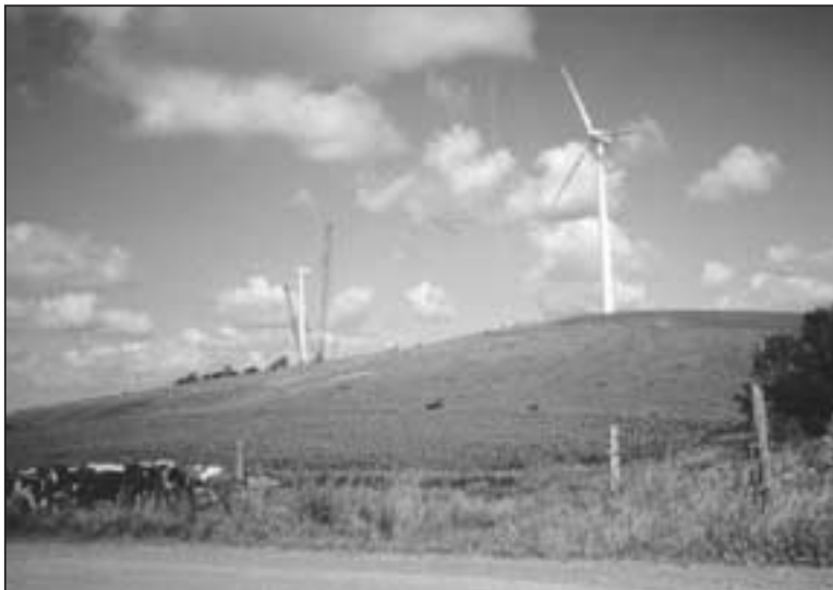
Figure 2.1 View of Fenner wind farm.
