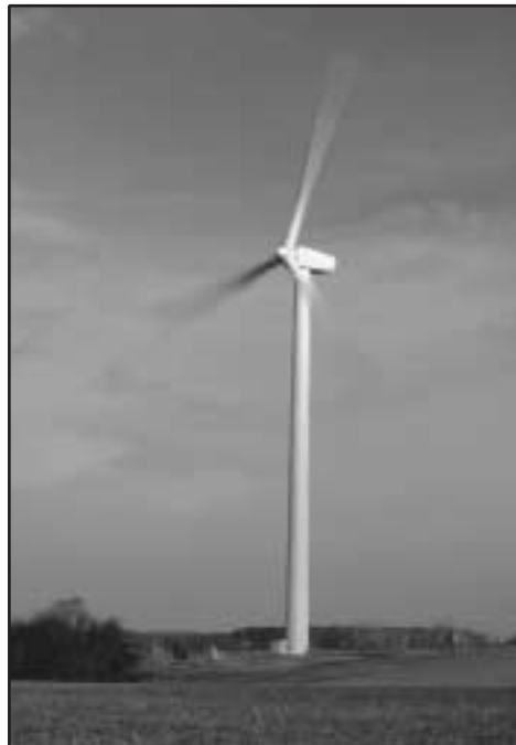
FIGURE 6.1 SOMERSET WIND TOWER
