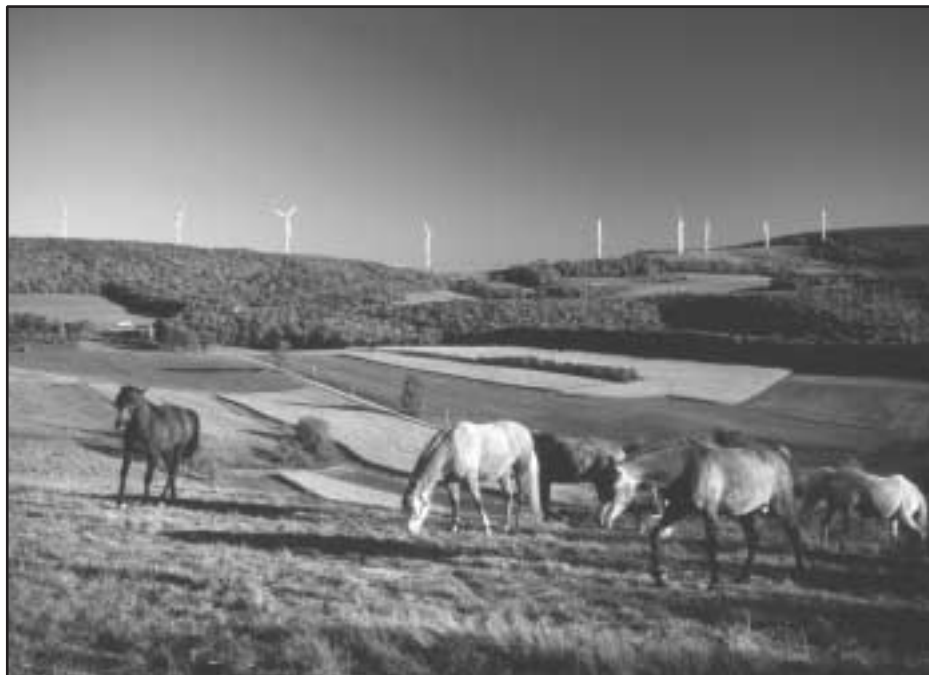
FIGURE 9.1 VIEW OF A MILL RUN TURBINES PHOTO COURTESY GE WIND ENERGY © 2002
